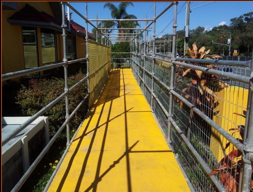
Figure 6 - Temporary Pedestrian Structure
